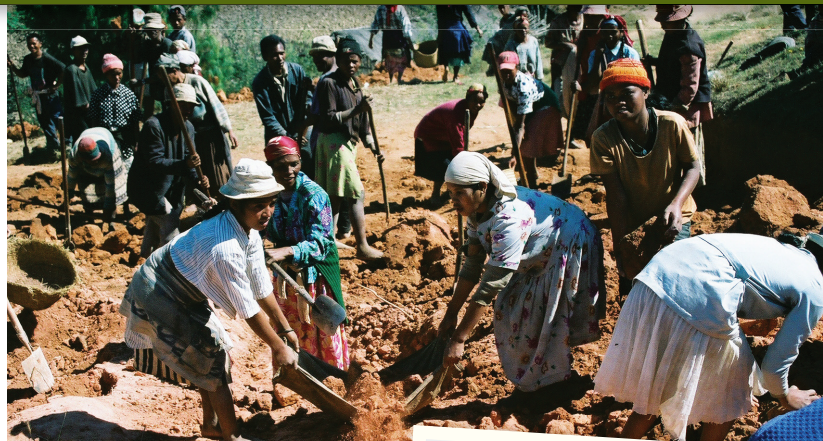
► Above: Women remove dirt that has been loosened with a spade by the men as the whole village, near Ansirabe, cooperates to lower the grade on their access road, making it easier to transport products in wet weather.
